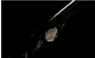
Scratched or chipped paint
