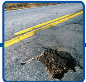
POTHOLE/DAMAGED PAVEMENT
