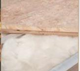
■ R-7 insulated floor with 5/8" tongue and groove exterior grade plywood on aluminum floor joists is standard. Competitors typically use OSB or particle board
