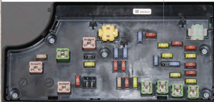
#13 Fuse 20 Amp Yellow – Power Outlet/Cigar Lighter Instrument Panel
