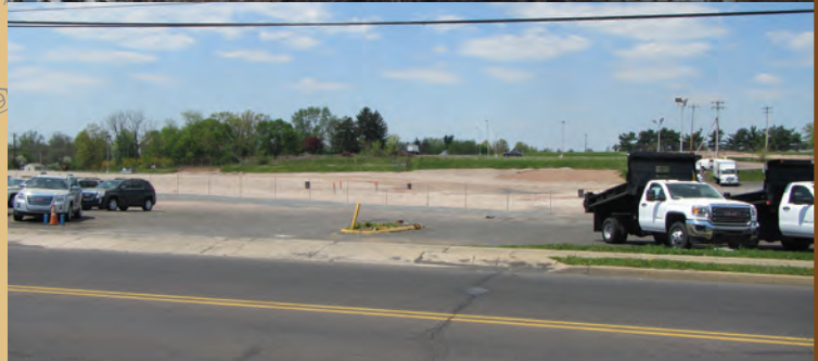
Stages of removal of building and clearing of site for new Franconia building
