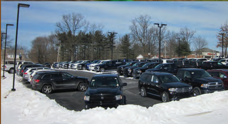
Completed CJD parking area
