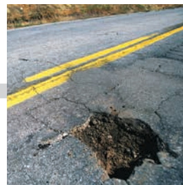
POTHOLE/DAMAGED PAVEMENT
