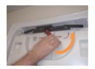
Step 10: Using the electric screw driver with Phillips head bit, fasten the four (4) screws into the holes in the receiver. Tighten each until the screw is fully seated. **Do Not Over Tighten Screws**
