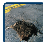
POTHOLES/ DAMAGED PAVEMENT
