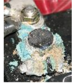
Corroded battery terminal end
