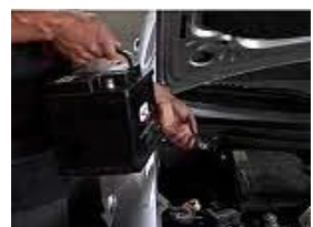
New battery installed by a trained technician
