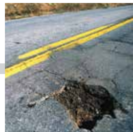
POTHOLES/ DAMAGED PAVEMENT
