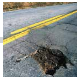
POTHOLE/DAMAGED PAVEMENT
