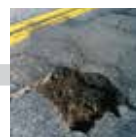
POTHOLE/ DAMAGED PAVEMENT
