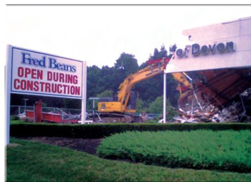
Making way for the new store
