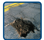
POTHOLES/ DAMAGED PAVEMENT
