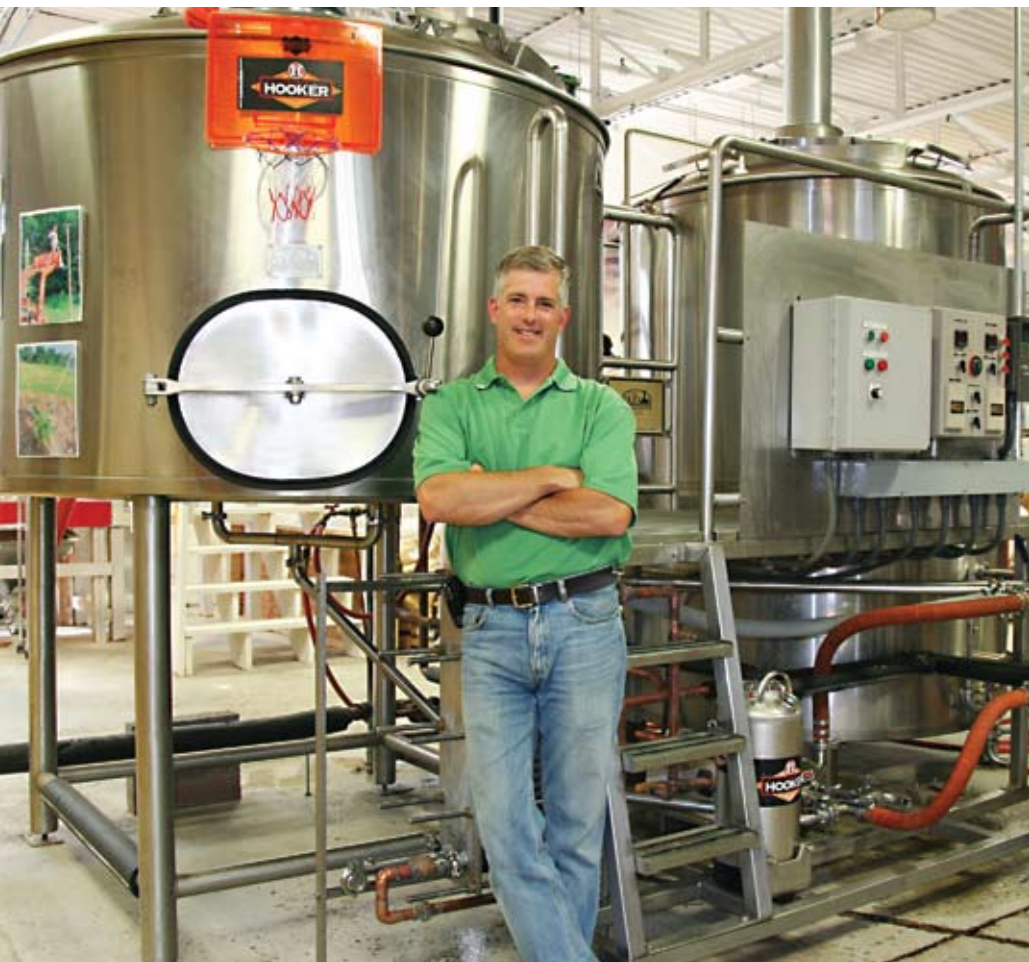
Curt Cameron, president of Thomas Hooker Brewery, looks forward to completing a major expansion that will double brewing capacity.
