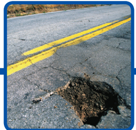
POTHoles/DAMAGED PAVEMENT
