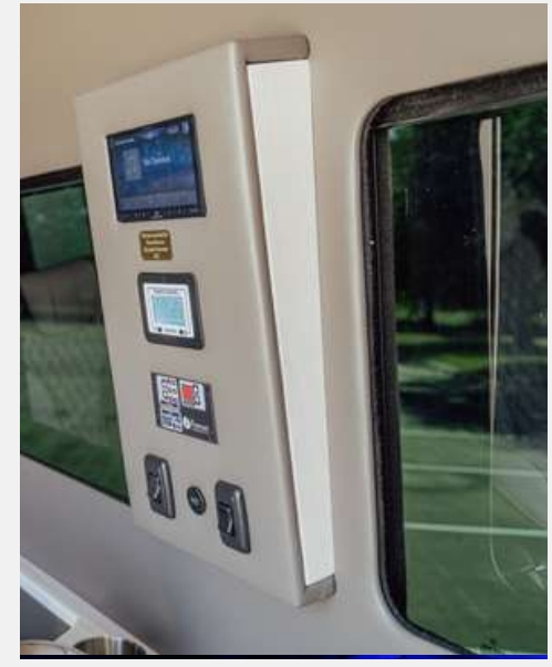
A/C & Inverter Control Panel
